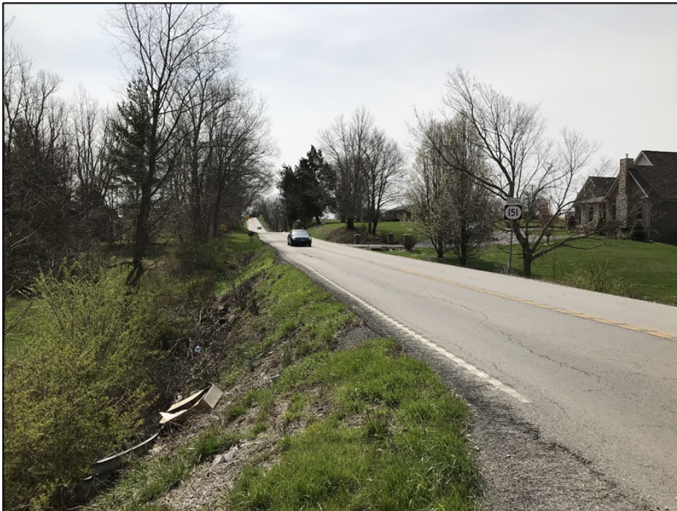
Figure 6: Steep slopes south of KY 2820
