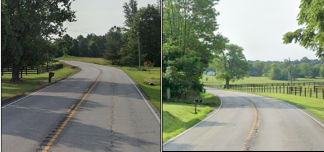
Figure 5: Horizontal Curves near Lin Moore Rd.
